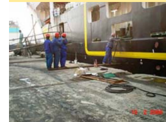
These four sure didn't take our scaffolding training!
